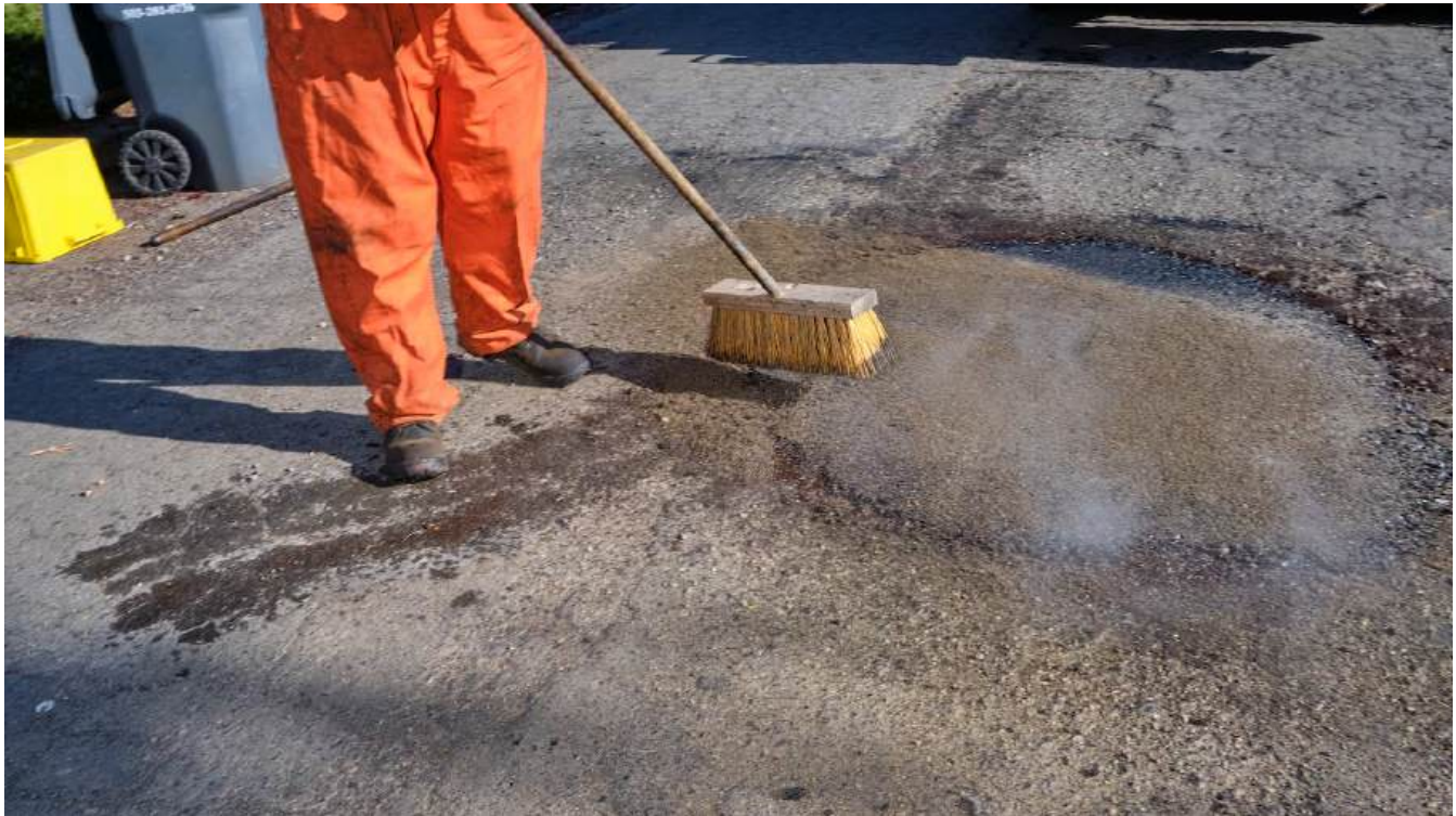
Portland Bureau of Transportation crews fill potholes. (Chris Nesseth)
